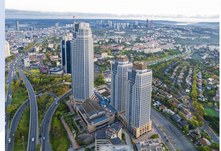
İş Towers Complex
